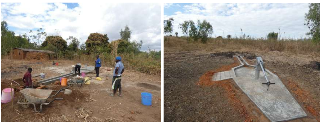
Pictorial presentation: Left- Civil works progress in Nsenda village and Right-Completed borehole in Maliwata Village.
