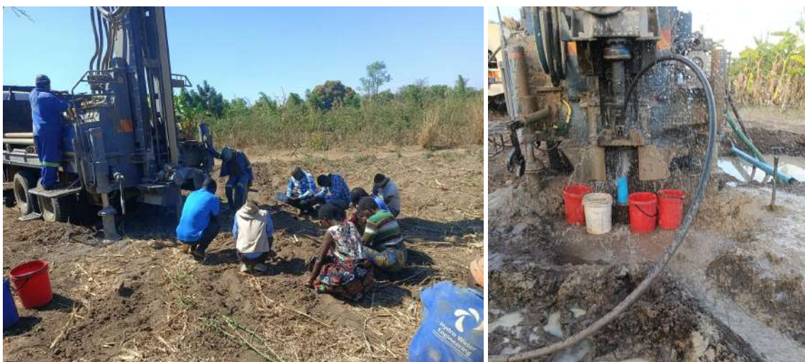
Pictorial presentation: Left-Community members praying before commencing drilling of a borehole on the second site of drilling in Makuluni Village and Right-Borehole development in progress in Makuluni Village after a successful drilling
